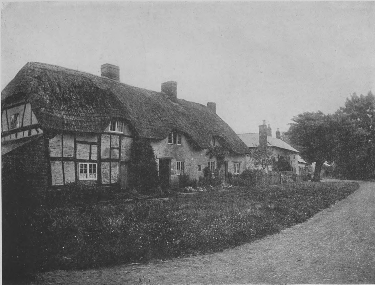
COTTAGES AT QUINTON IN WARWICKSHIRE
